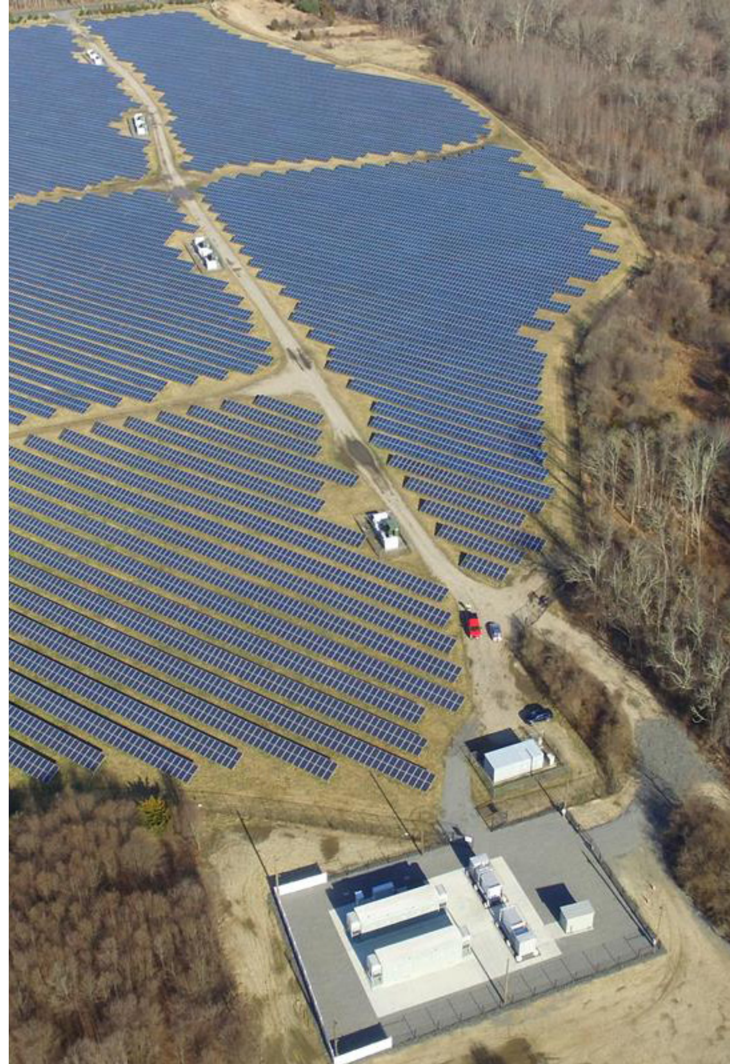
Howell, NJ, U.S., 7 MW \ 7 MWh
