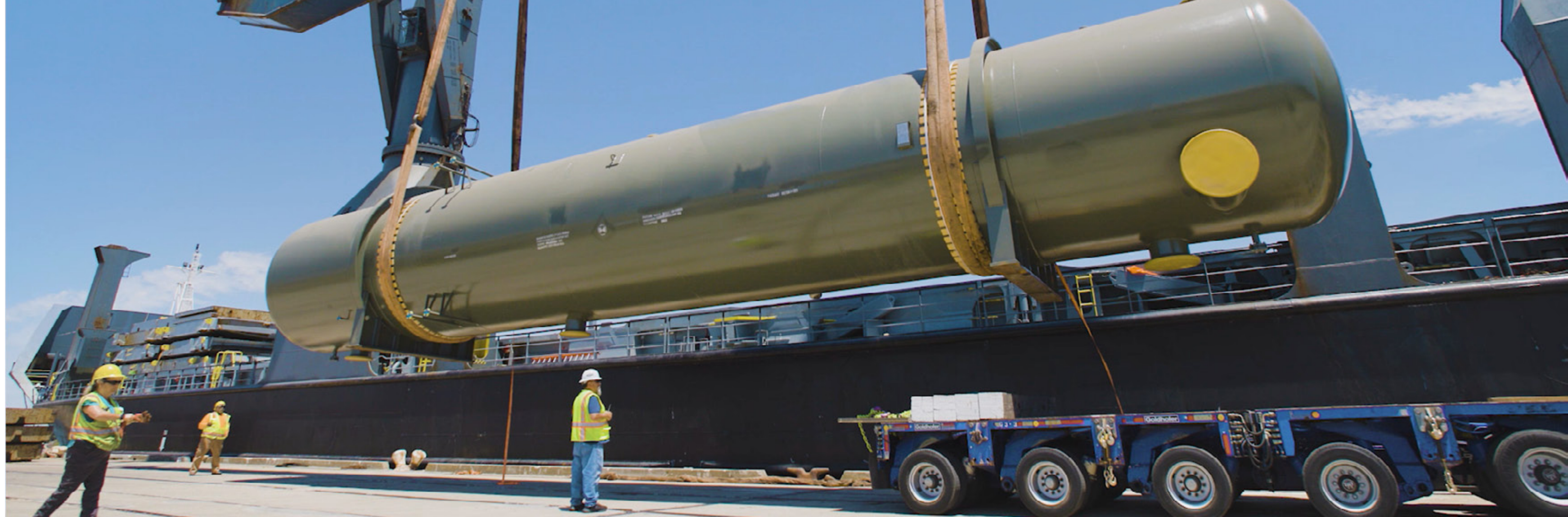
CD4 Power Plant constructions
