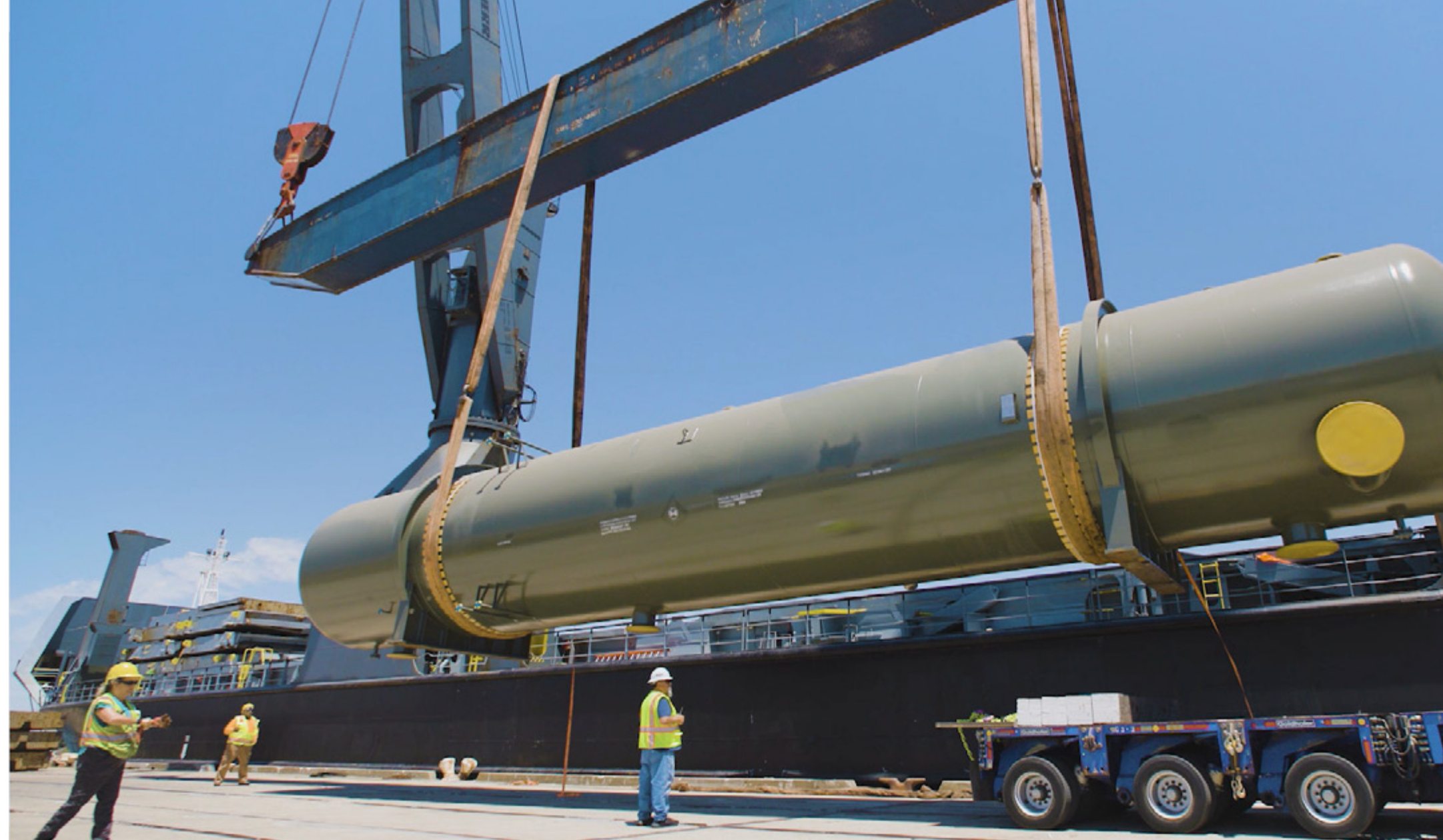
CD4 Power Plant constructions
