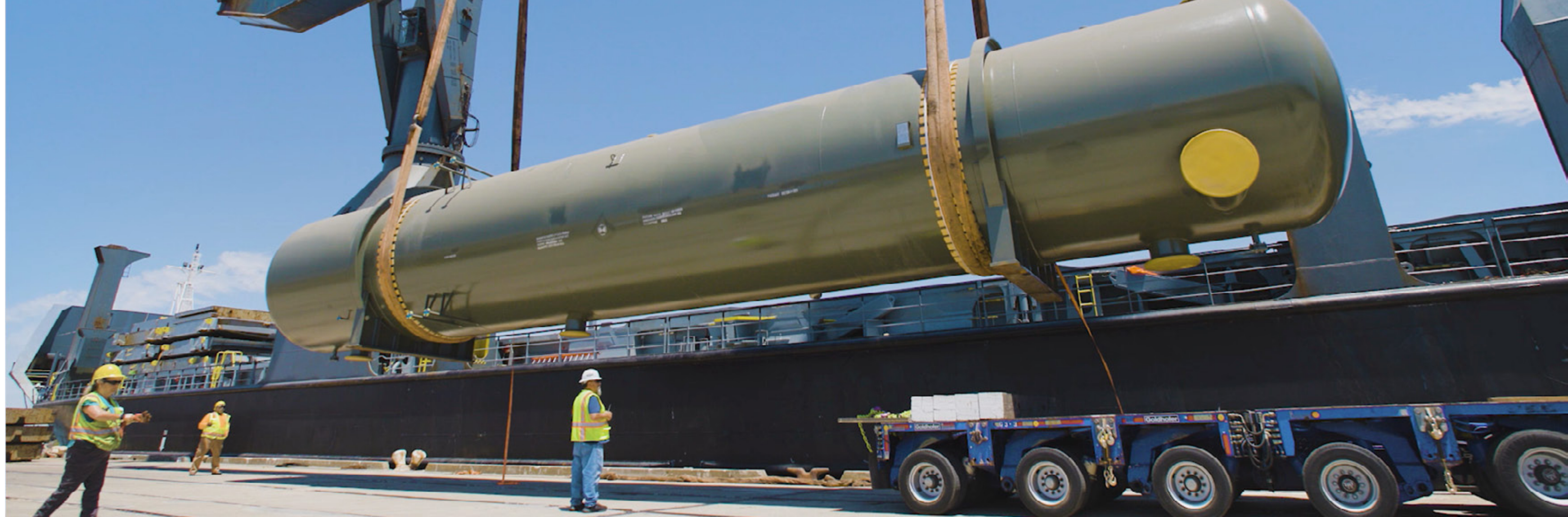
CD4 Power Plant constructions
