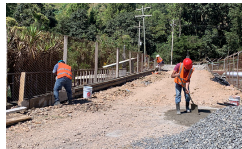
Supporting Bridge Improvement Work in San Jose Calderas Village, Ortitlan
