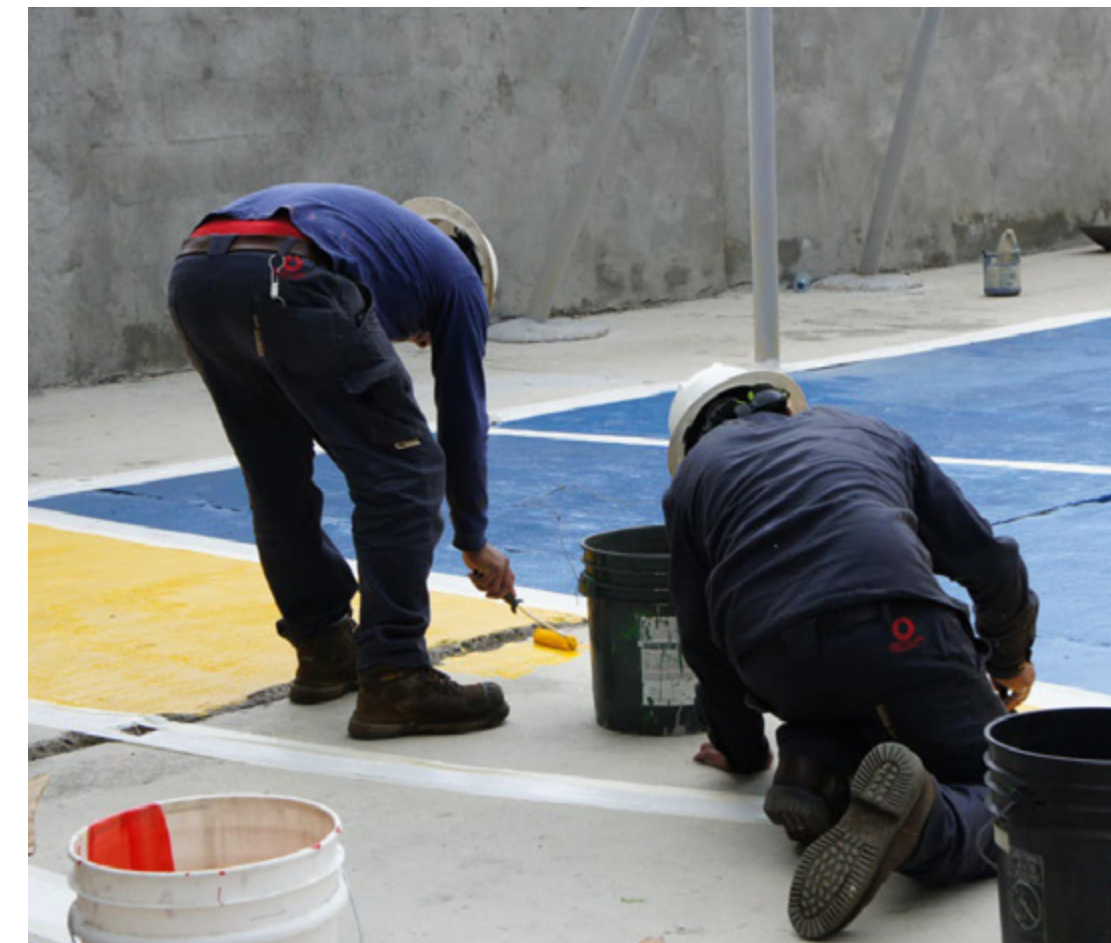
Renovation of a public basketball court, Ortitlan employees, Guatemala
