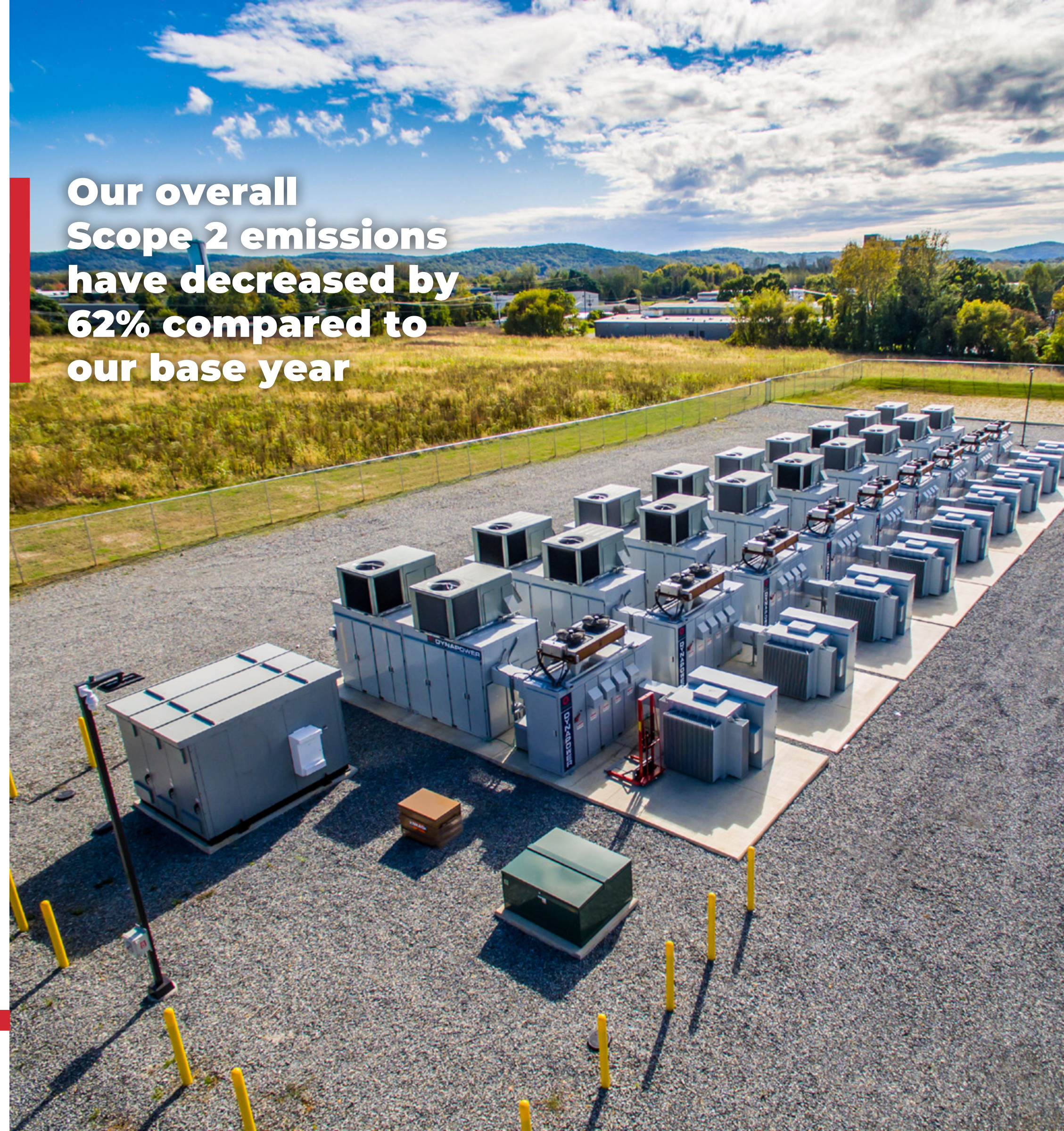
Stryker Alpha storage facility, NJ, U.S., 20 MW / 20 MWh
